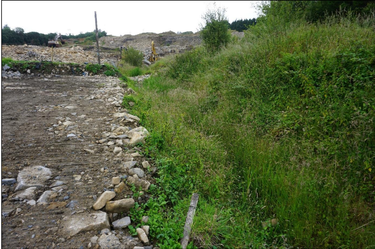
Photograph 8.1: Impeded pathway for site discharge to tributary of Eany Water
